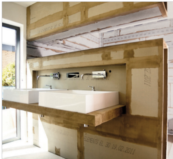
■ Two construction panels with different requirements are used for the intermediate wall. The factory-sealed and vapour-barring product LUX ELEMENTS®-ELEMENT-VK was used in the rear shower area.
