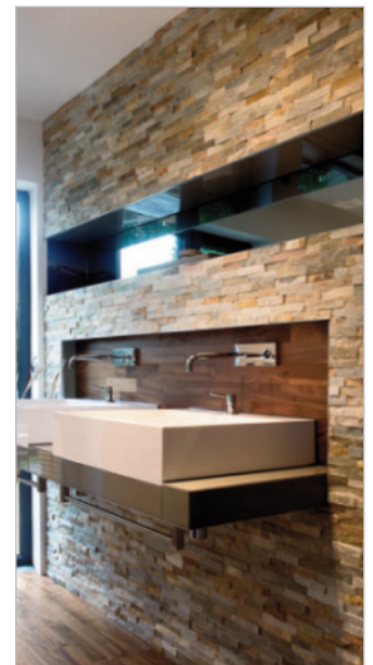
■ After completion – the white design washstands made of elegant cultured marble form an attractive contrast to the natural stone strips.
